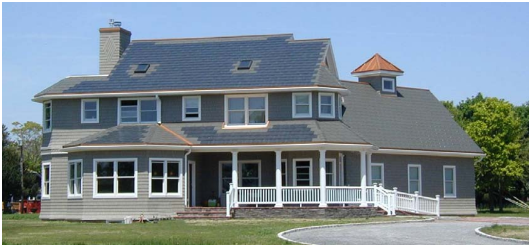
10 kW SUNSLATES™ System over 15 kW Dawn Solar System
